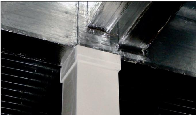
Figure 1. Fire protection boards – decorative (white) boards on the columns and non-aesthetic (silver) boards on the beams
