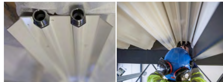
Fig.1 Ruukki radiant panel and installation
