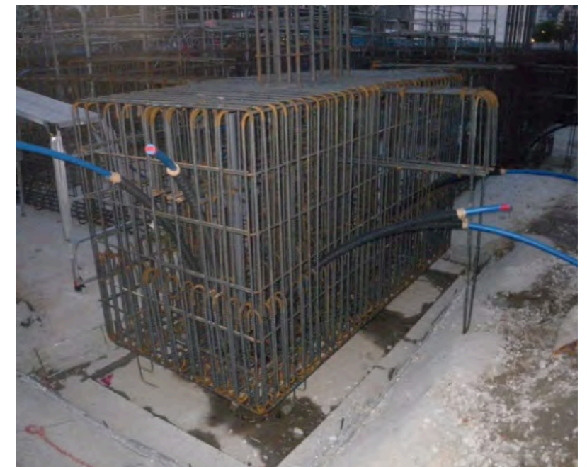
Fig.6 Remove U-tube from footing in specified directio
