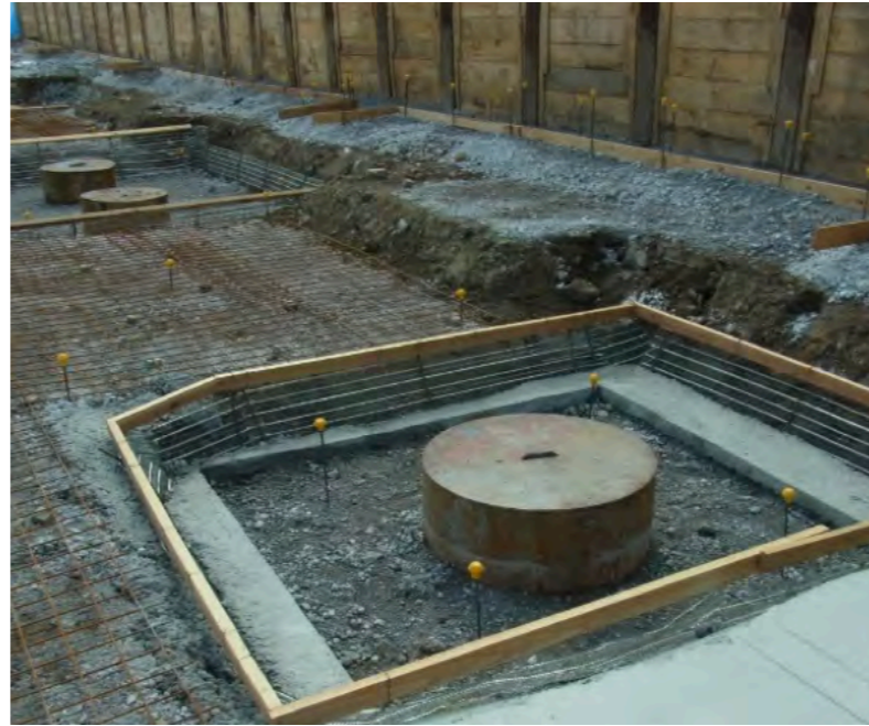
Fig.3 Pile head after penetrating steel pipe pile (after attaching curing lid)
