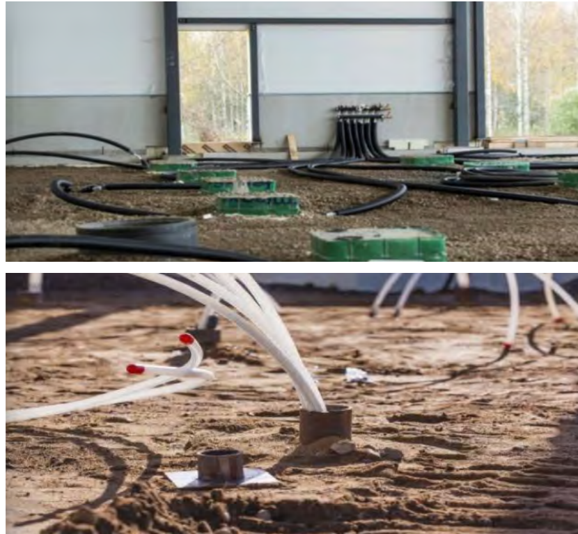
Fig.3 Heat collector pipes installed in the floor slab pile
