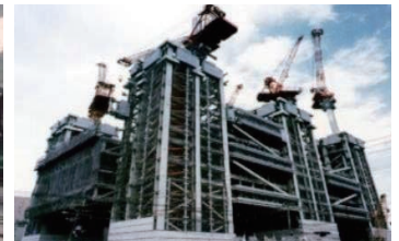
Buckling-restrained brace
