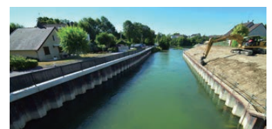
River protection, Fouchy a Troyes, France
