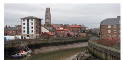
Boston Barrier Flood Defence, Boston, UK
