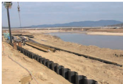
Cutoff wall for river embankment
