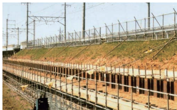
Example of embankment railway
