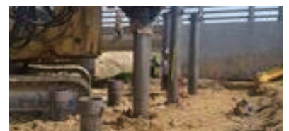
Osung IC pier, Pyeongtaek
