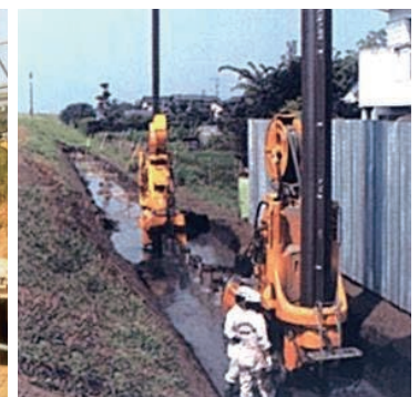
Example of press-in pile driving
