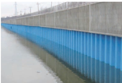
Kyung-in Canal Shore Protection
