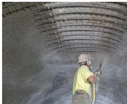
2.Tunnel and culvert shotcrete lining
