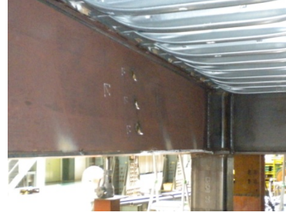
(b) Appearance around the studs
