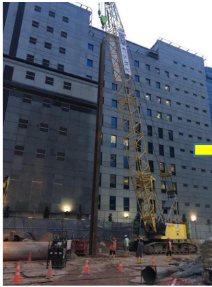
(a) Installation of King Post
