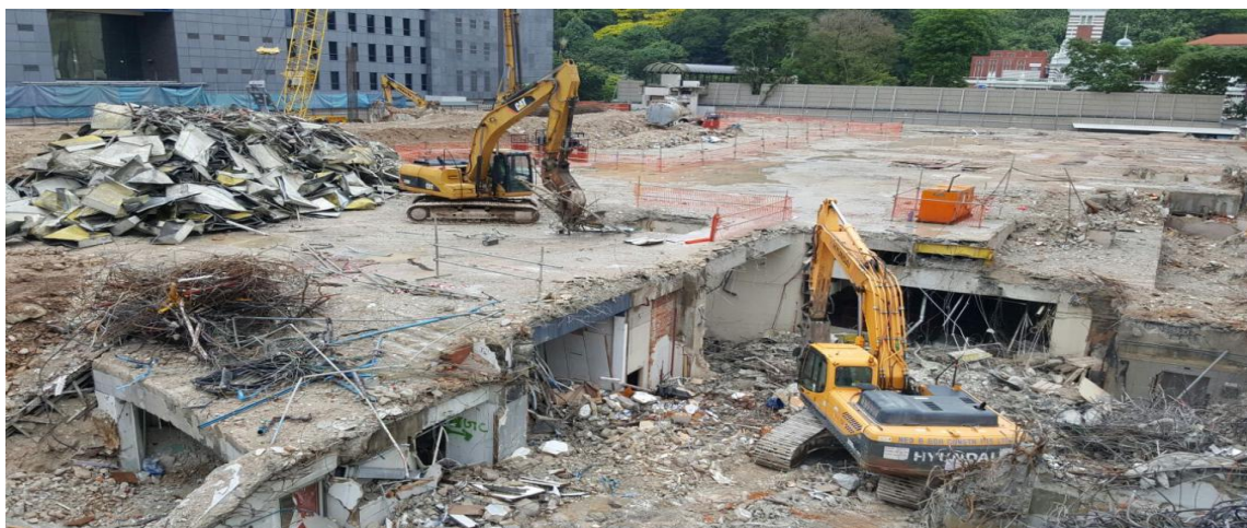
Figure 2. Site condition with existing basement structures during Site Possession
