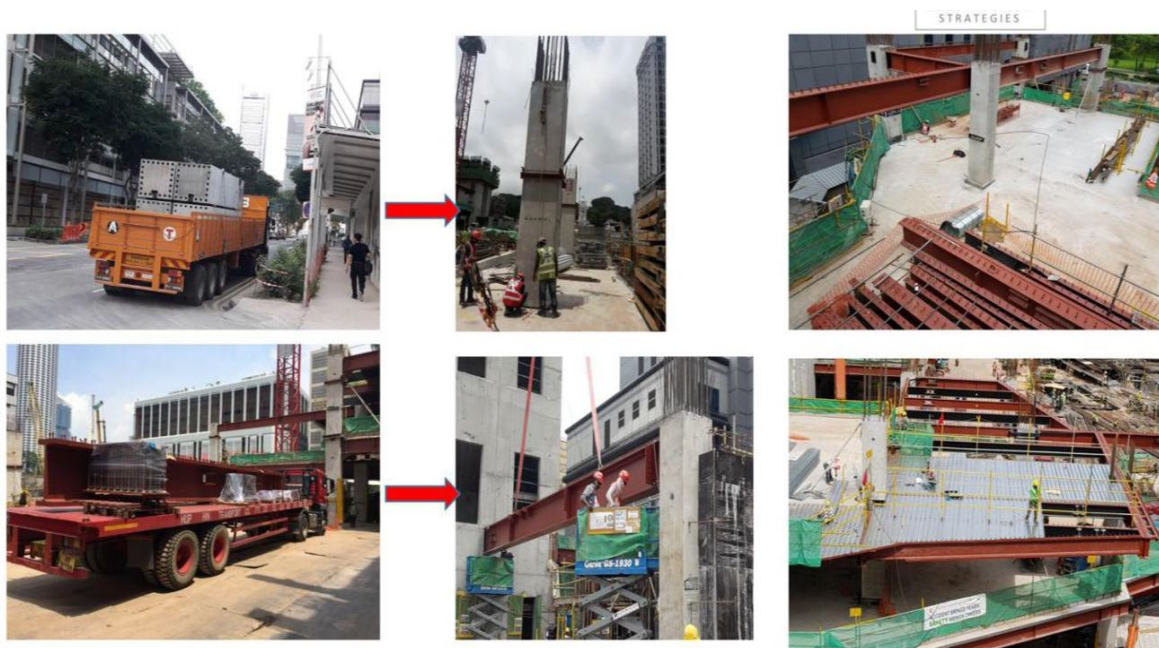
Figure 6. Work Flow of the Hybrid System
