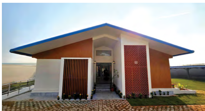
Figure 26. The Zero Energy Building, Bhubaneswar, India – front view. © TataSteel & constructsteel
