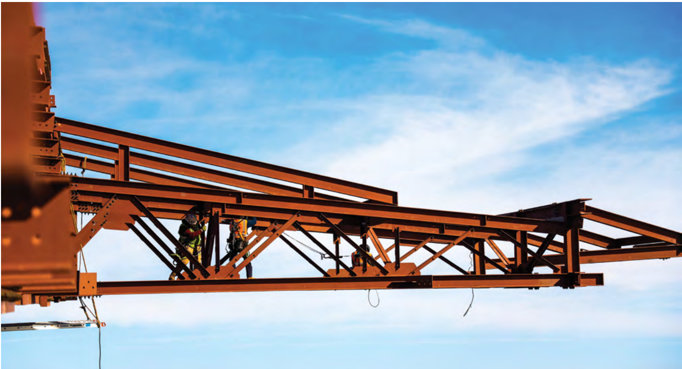
Figure 10. Cantilevered truss during construction. © Matt Good
