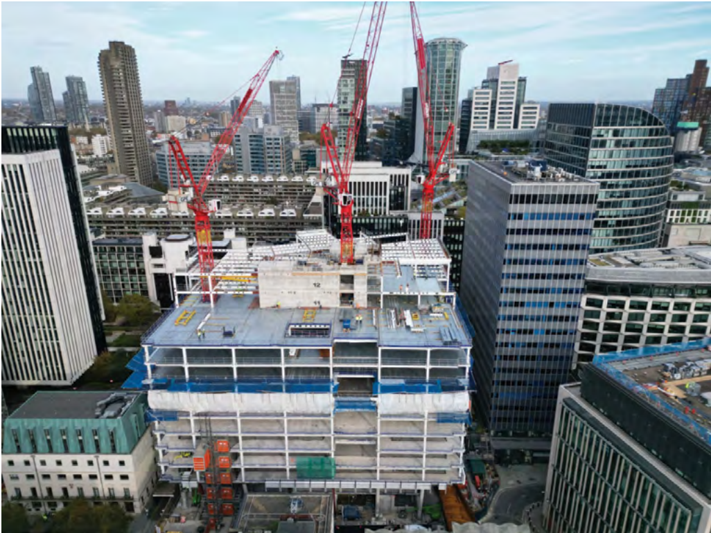
Figure 8. 2 Aldermanbury Square, London – under construction. © Bovis
