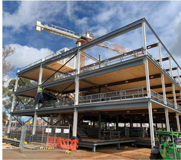
Figure 17. St. Marys Integrated Project Office (IPO), Sydney, during construction. © Joseph Bonica, RBG
